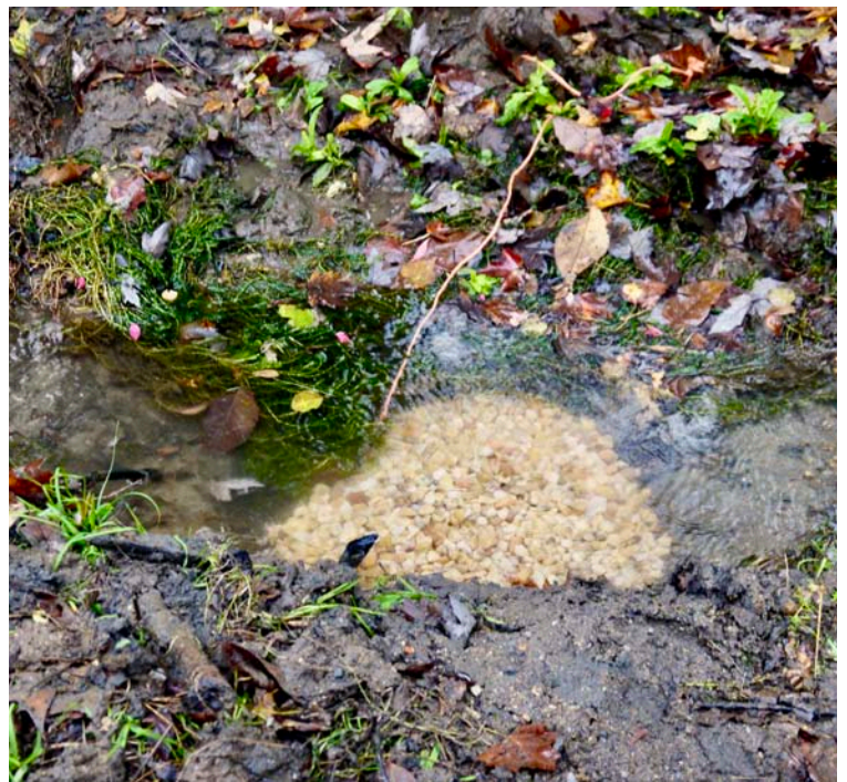
Box Covered By More Washed Gravel. Orange Finder Line Set For Spring Check Up
